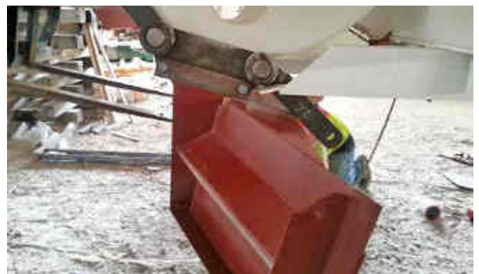
Installation of a shovel
