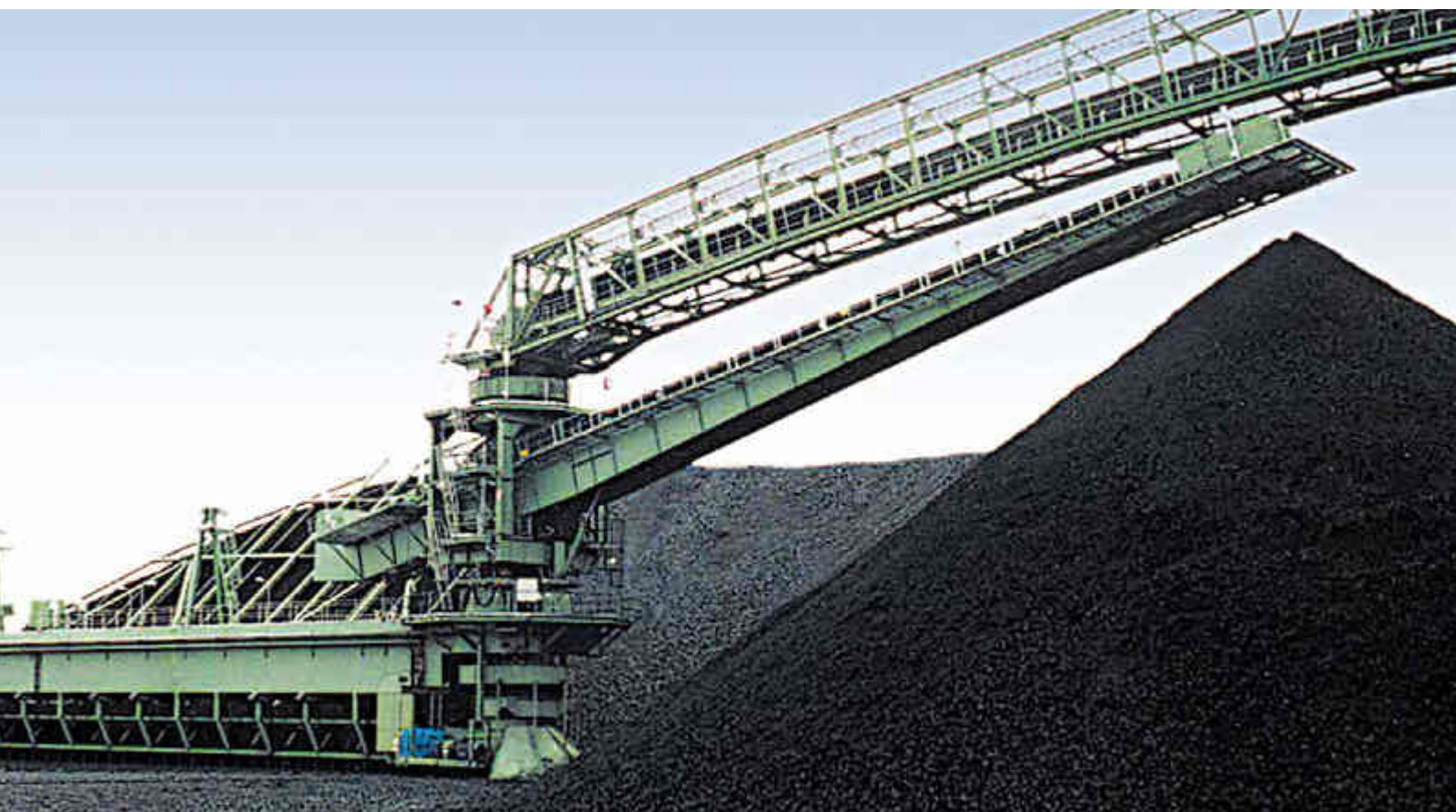
Circular Stacker / Bridge Scraper Reclaimer, rail dia 120 m, stacking 2,500 t/h, reclaiming 1,600 t/h, Coal
