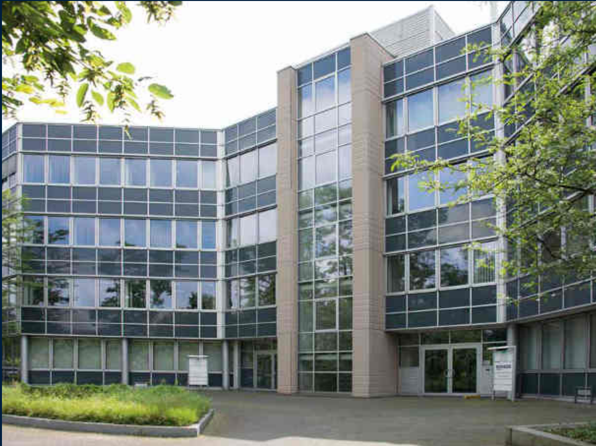
SCHADE Headquarters Gelsenkirchen, Germany
