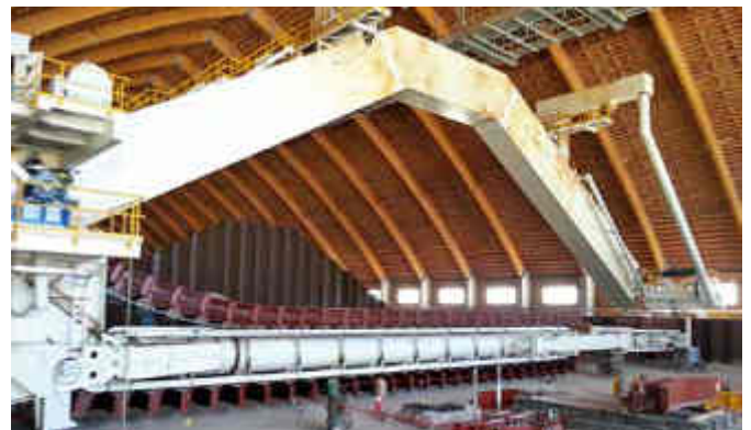
Erection of the portal by chain
