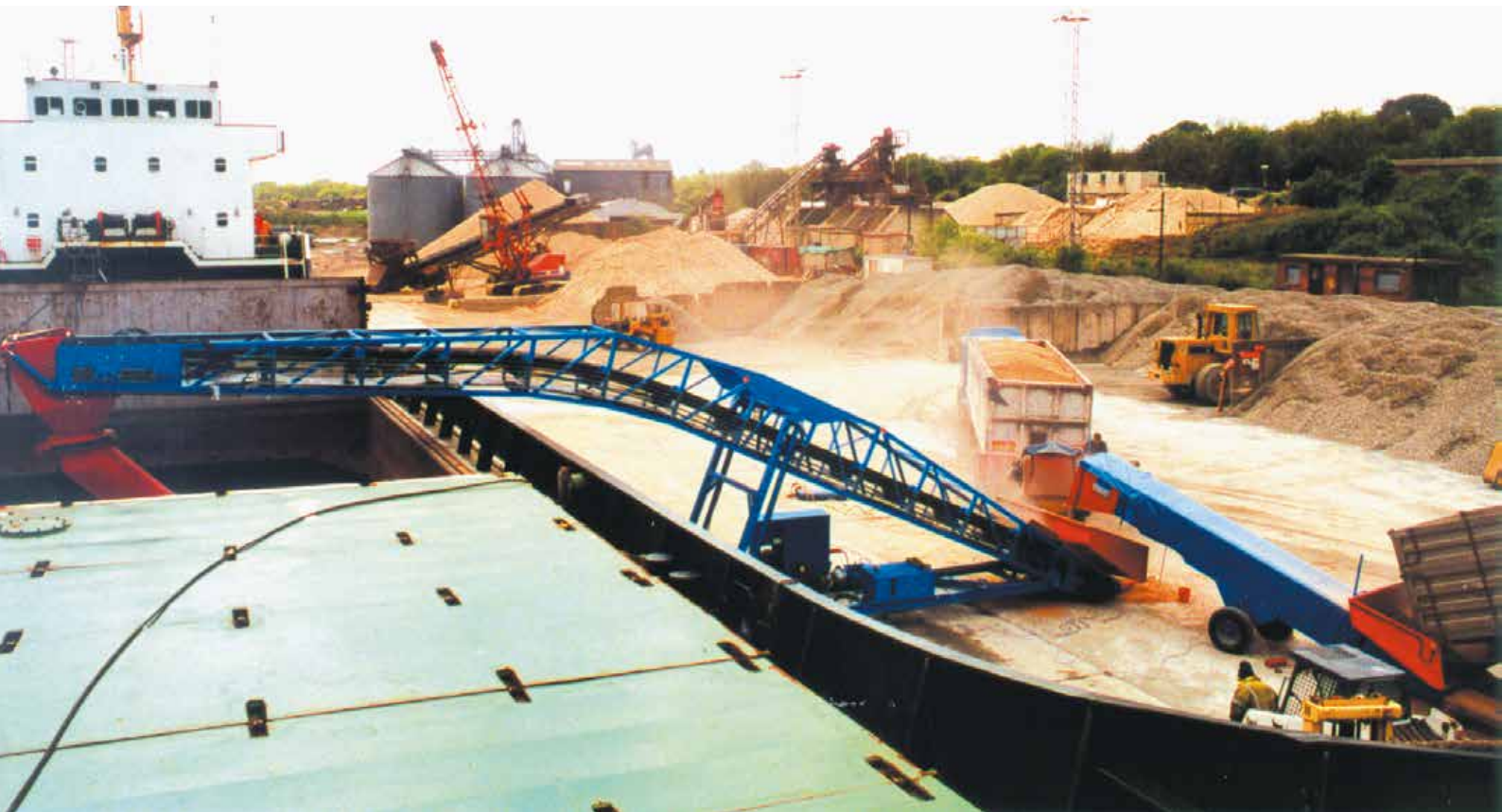
Feeder conveyors discharge to the Shiploader
