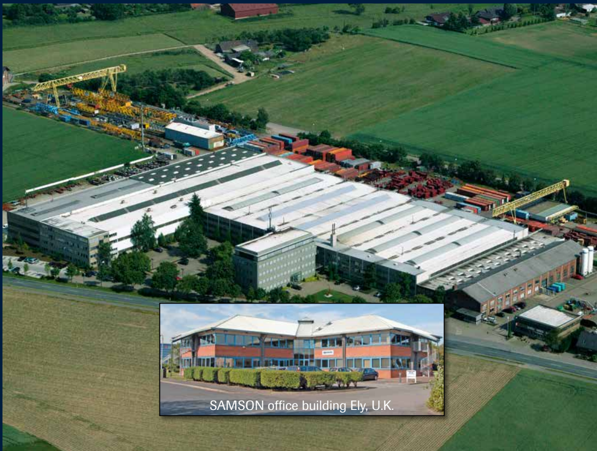
AUMUND GROUP Headquarters in Rheinberg, Germany
