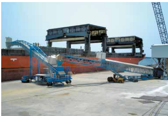
Shiploader – Conveyor Feed
