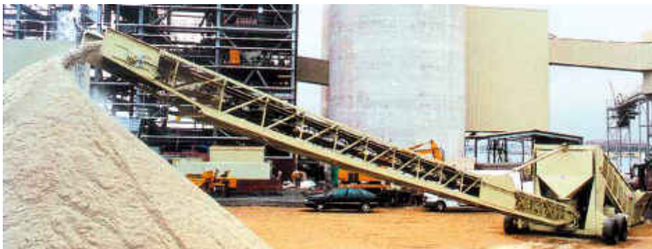
Stormajor® stockpiling granulated steel slag direct from tipping trucks
