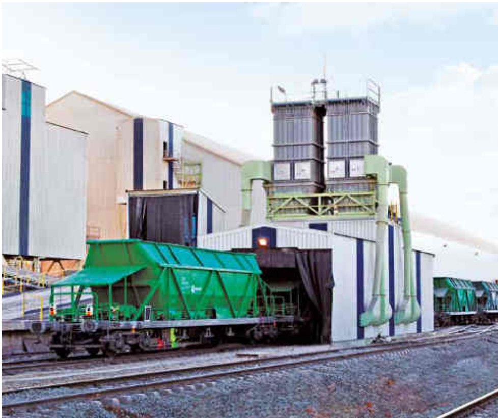
Discharge facility for hopper bottom railcars receives coal for a cement plant including a Samson® Material Feeder with 80 tons holding capacity
