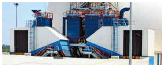
Twin Samson® side tip feeders with vertical elevators to dome storage
