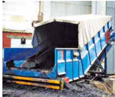
Flexible PVC sheet partial enclosure
