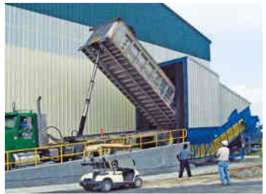
Synthetic gypsum intake to board plant
