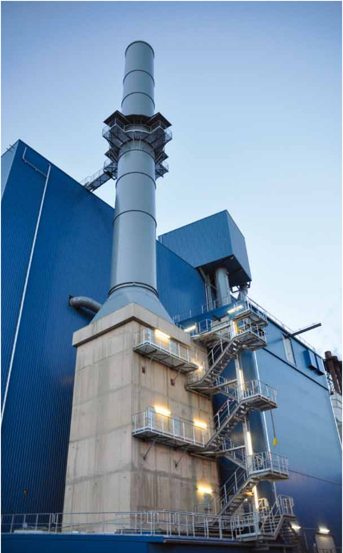
DEDUSTING PLANT FOR SAARSTAHL AG IN VÖLKLINGEN, GERMANY, COMMISSIONED 2012.
