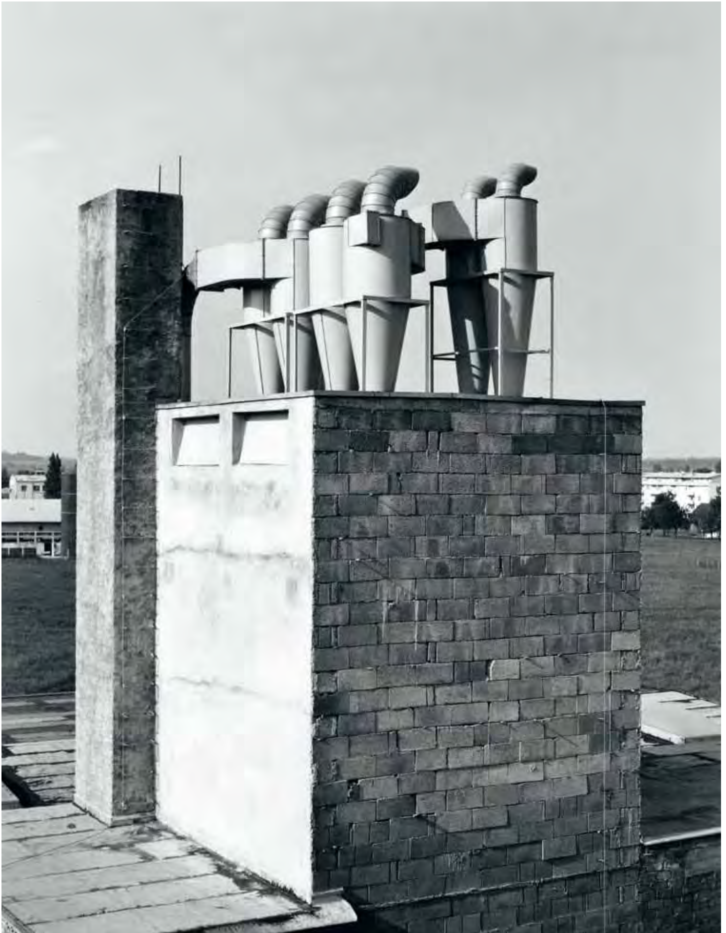
IN THE EARLY DAYS SCHEUCH USED CYCLONIC DEDUSTING.
