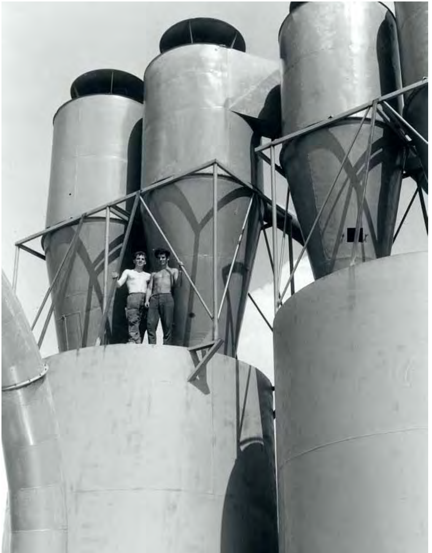
SOME ASSEMBLY WORKS WERE CARRIED OUT AT GREAT HEIGHTS.
