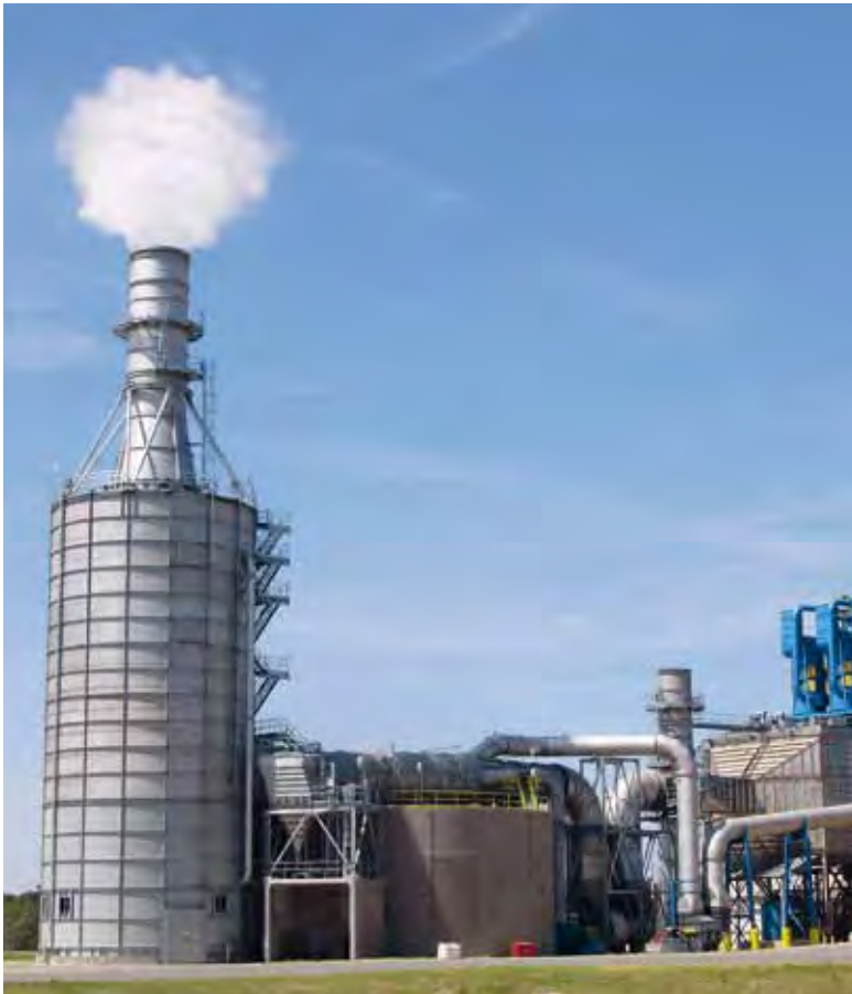
SCHEUCH IN THE USA: AT LANGBOARD IN WILLACOOCHEE, GEORGIA, IN 2009 A SABA BIOLOGICAL SCRUBBER IS DELIVERED.
