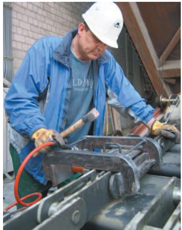
Pre-assembly of chain strands
