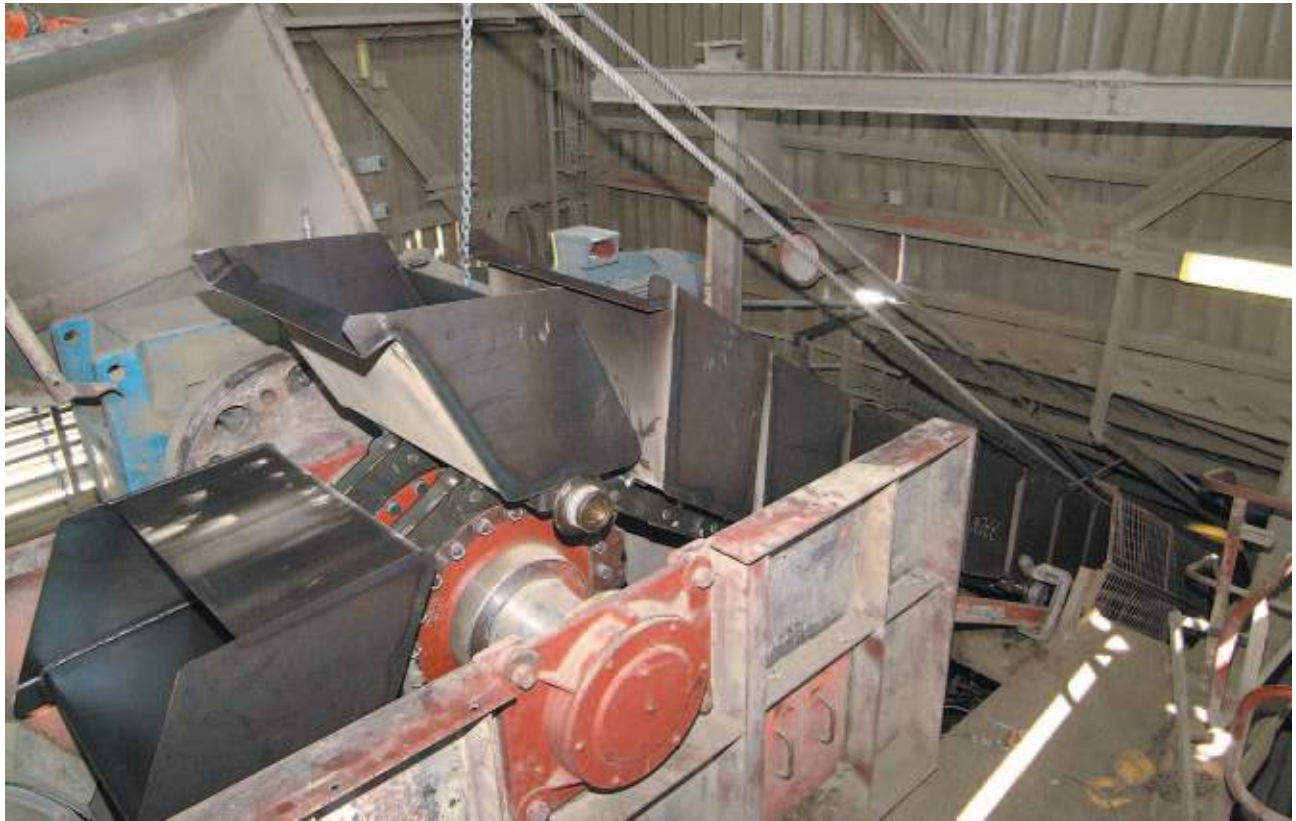
Installation of new bucket strand
