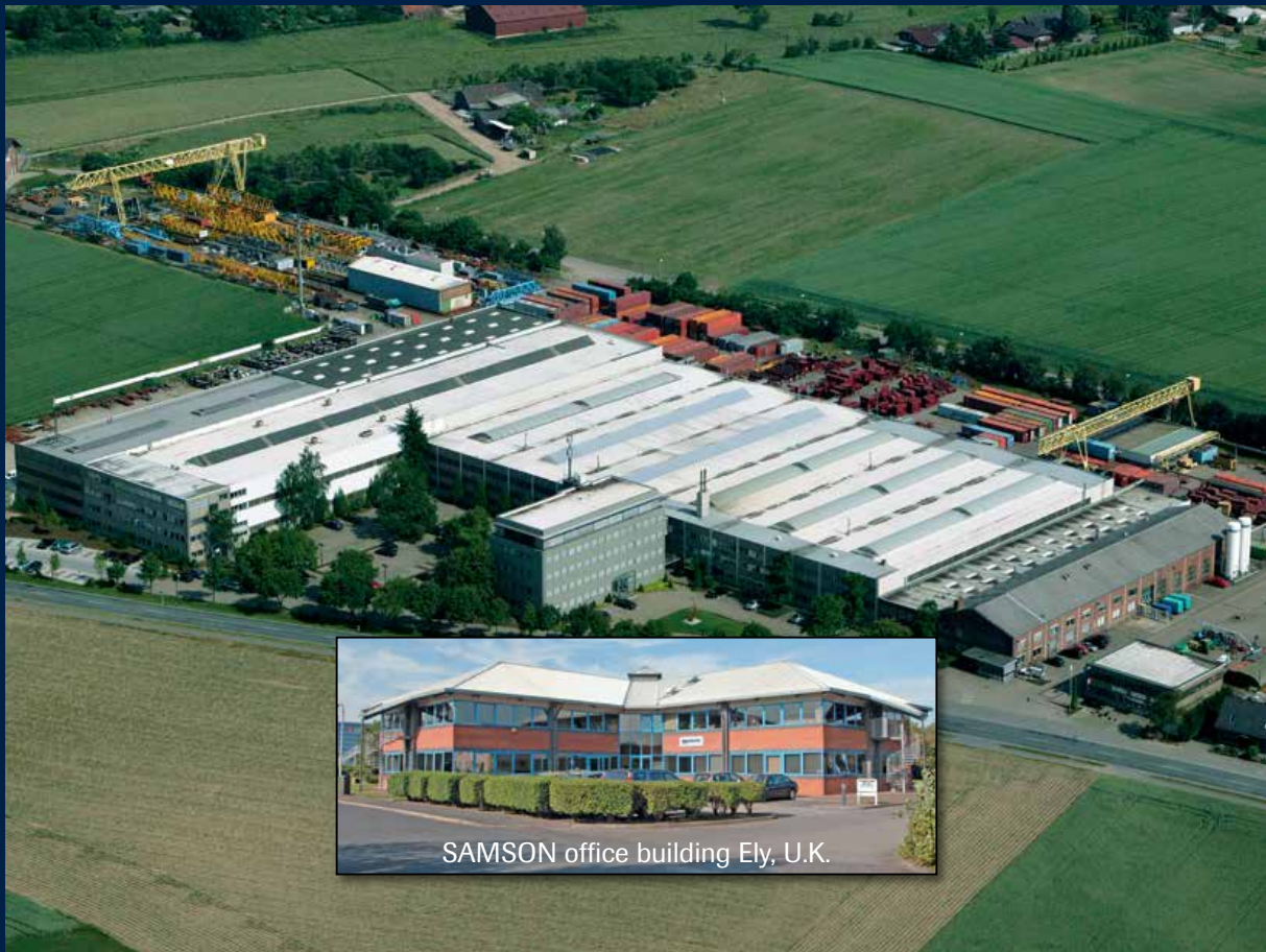
AUMUND GROUP Headquarters in Rheinberg, Germany
