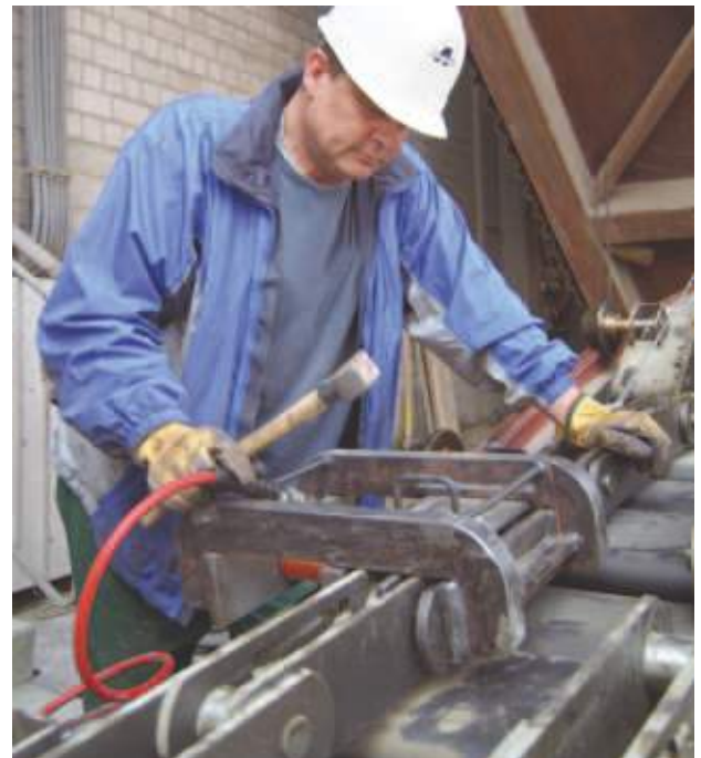
Pre-assembly of chain strands
