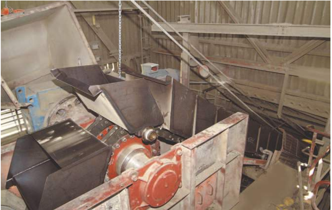
Installation of new bucket strand
