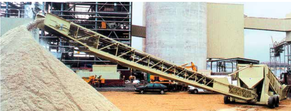
Stormmajor™ stockpiling granulated steel slag direct from tipping trucks
