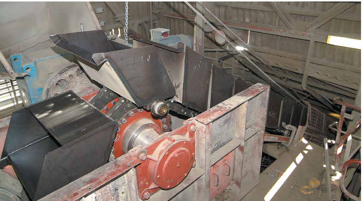
Installation of new bucket strand
