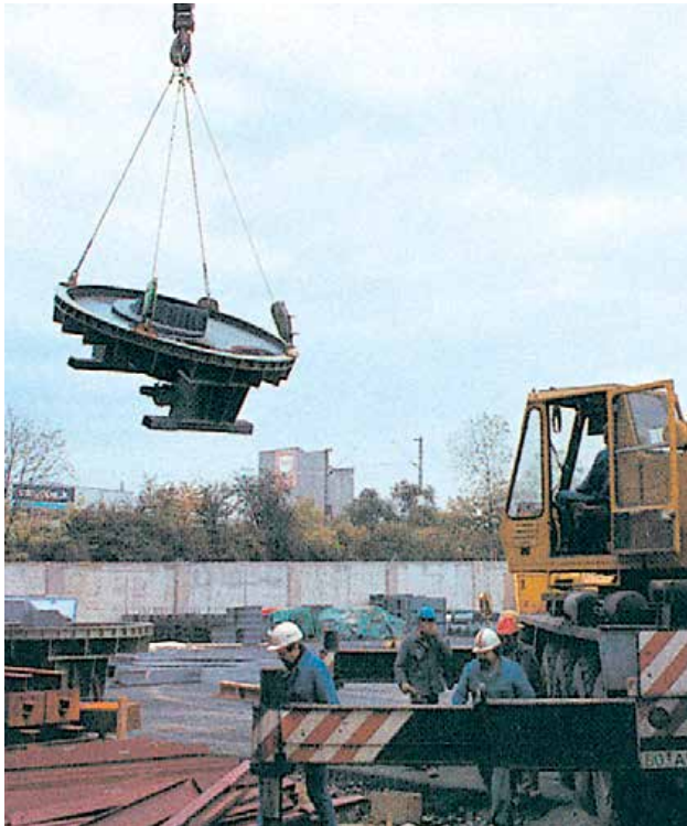
Lifting of workshop
