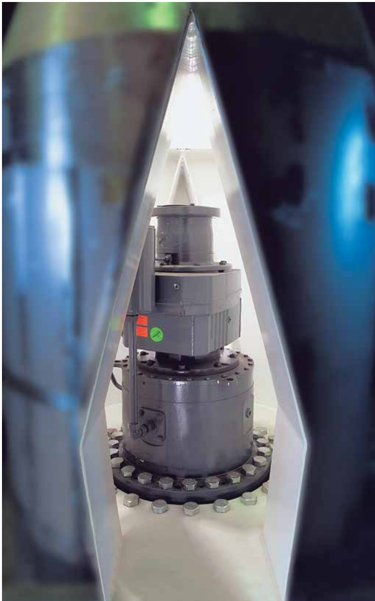
View through the hollow girder onto the drive unit
