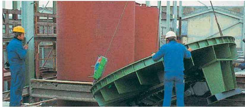
Assembling of CENTREX™ bottom in the field
