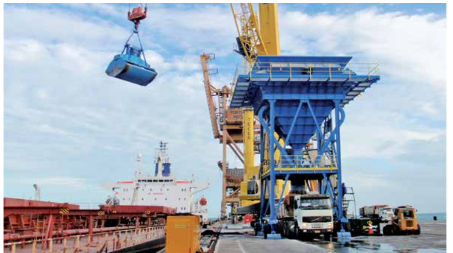
Truck transfer from Eco Hopper to inland storage
