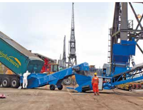
Independent Feeder Conveyor for flexibility on the berth
