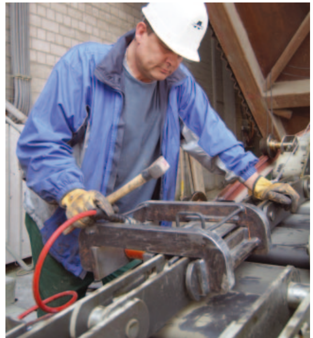
Pre-assembly of chain strands
