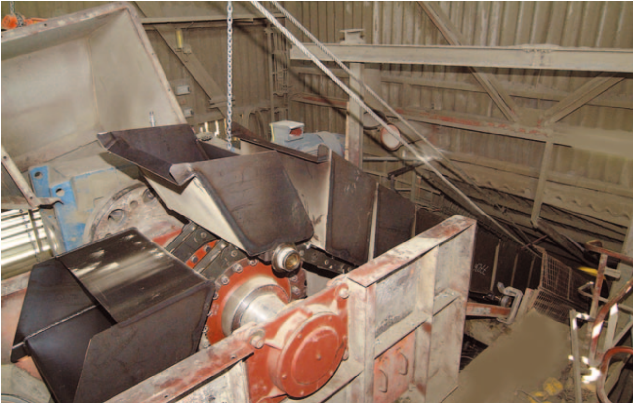
Installation of new bucket strand
