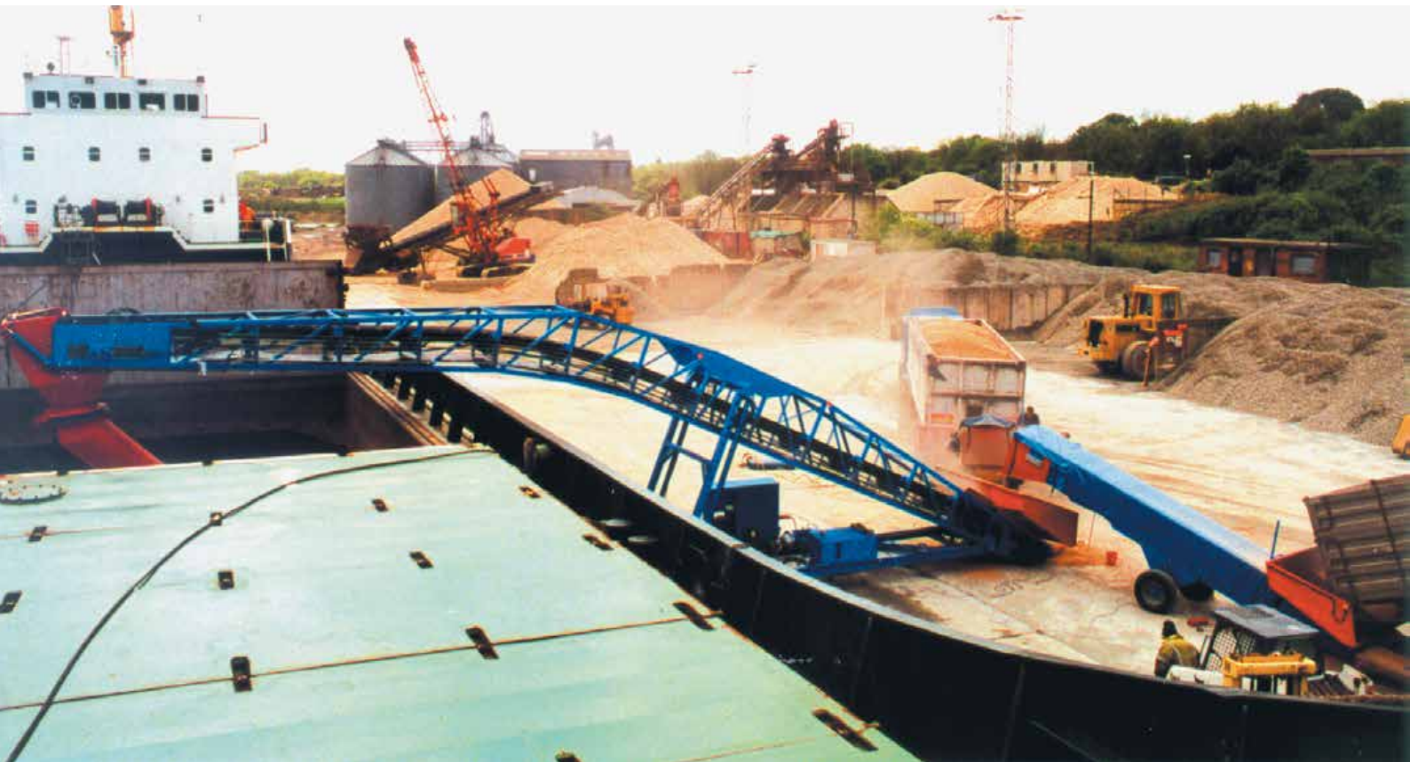
Feeder Conveyors discharge to the Shiploader
