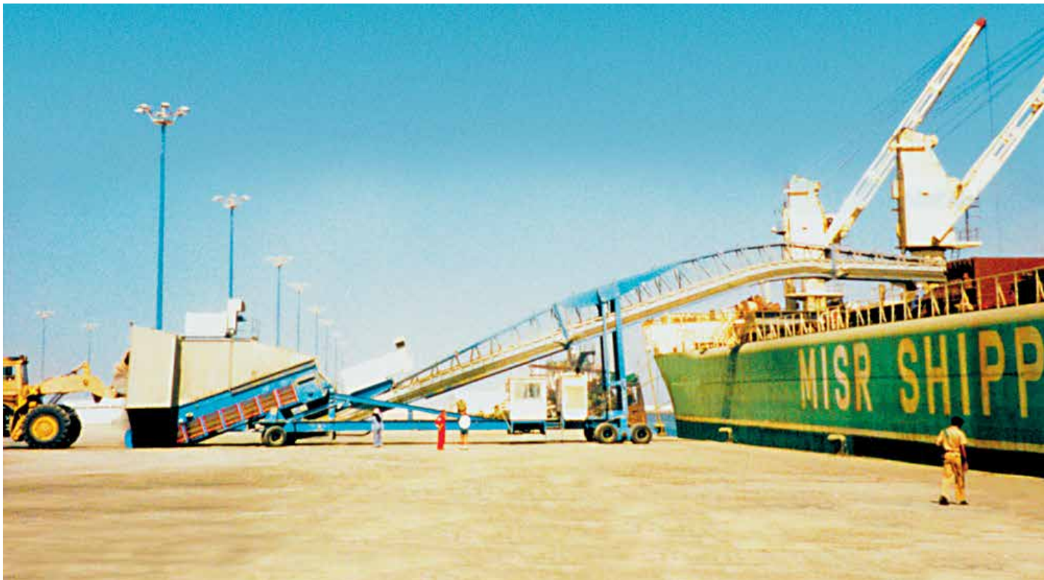
Full specification Shiploader handling Cement Clinker to Handy size ships
