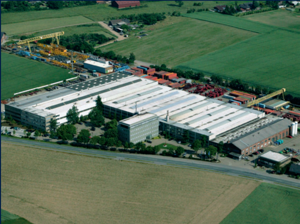
AUMUND Headquarters in Rheinberg, Germany
