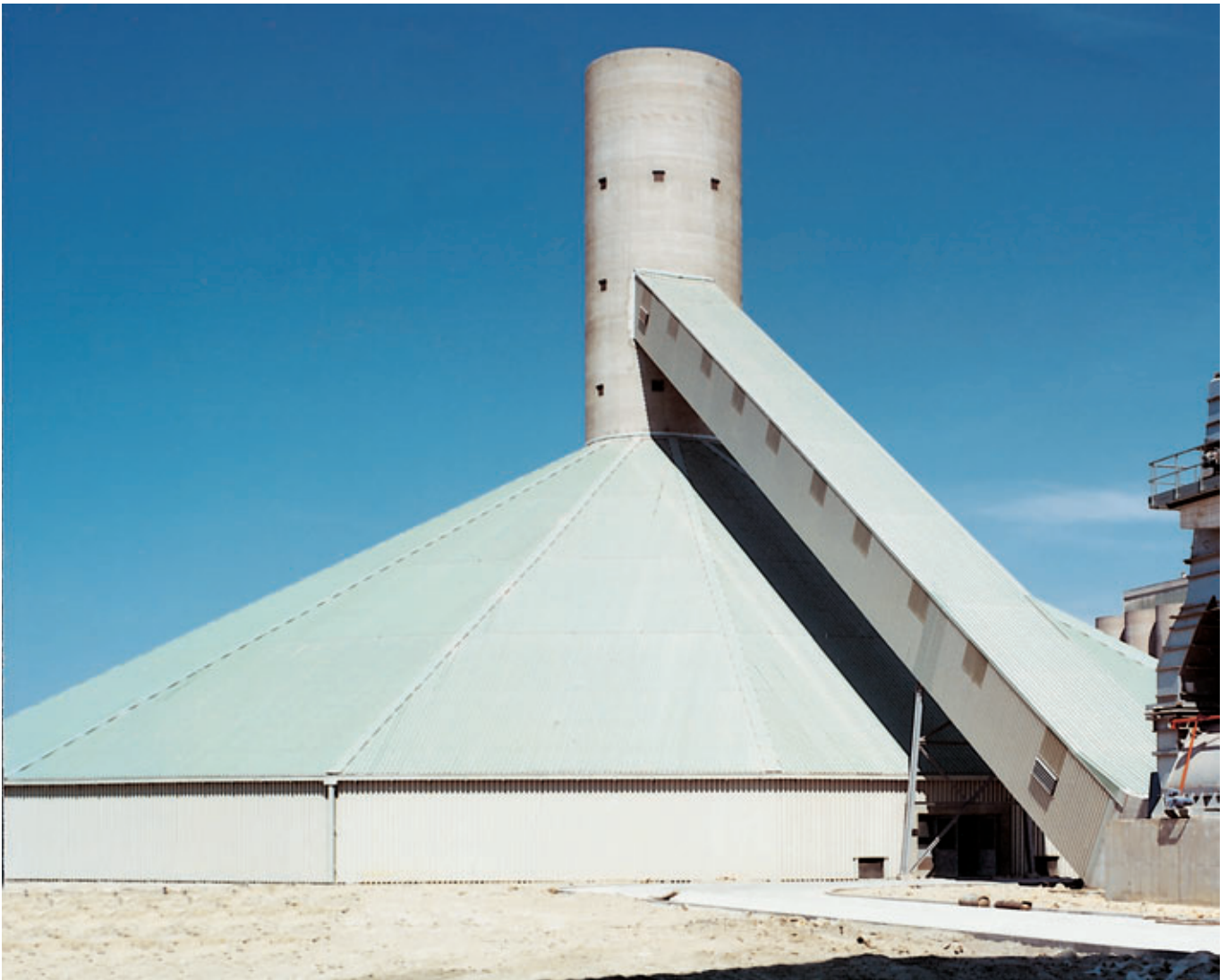
Feeding of covered stockpile
