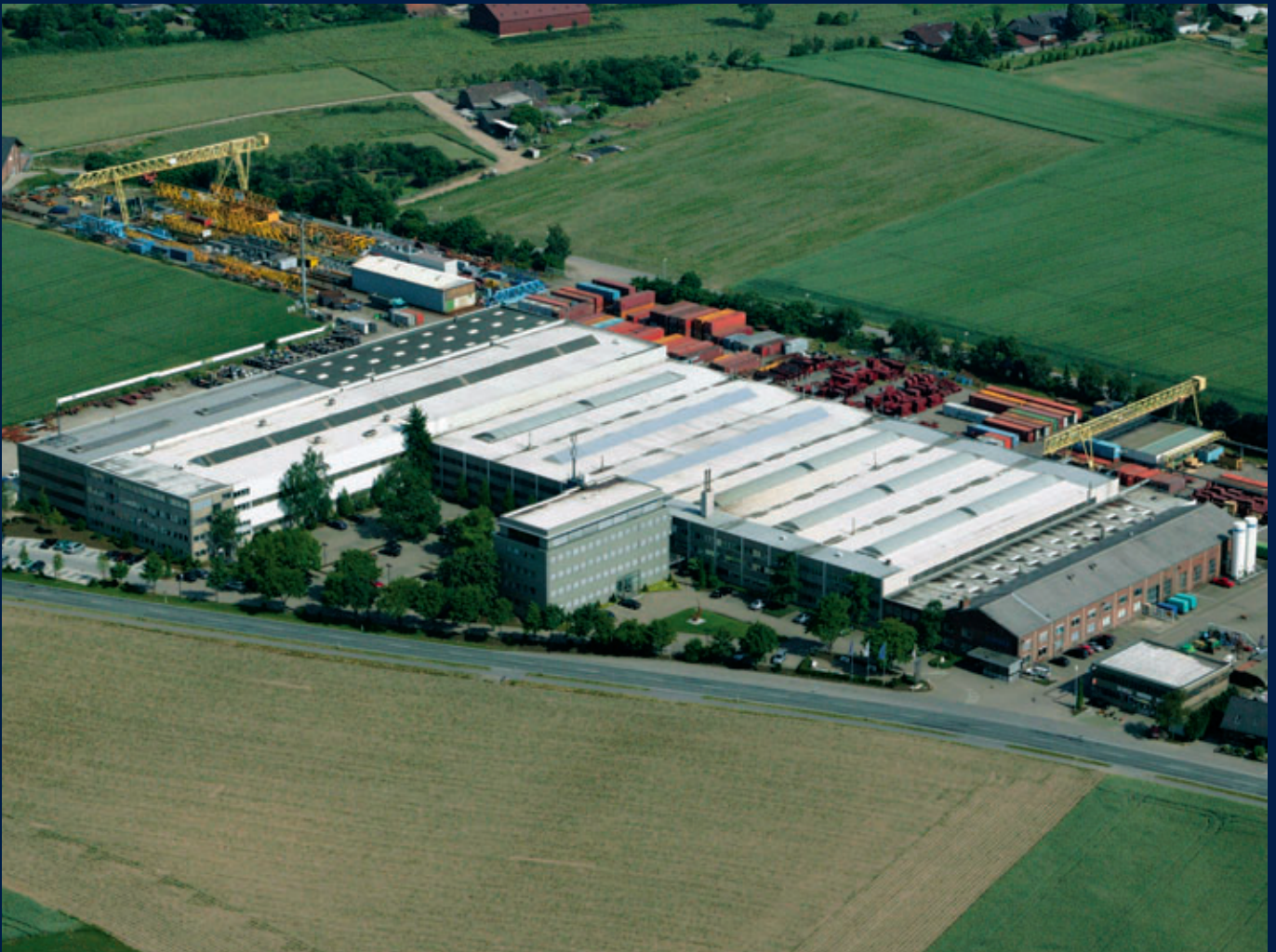
AUMUND Headquarters in Rheinberg, Germany
