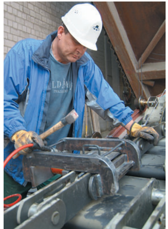
Pre-assembly of chain strands
