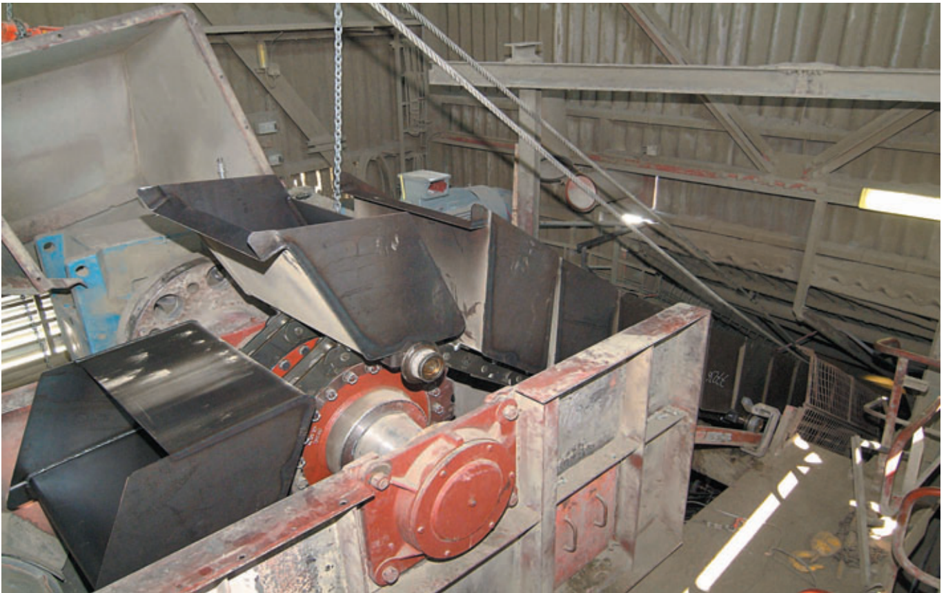
Installation of new bucket strand
