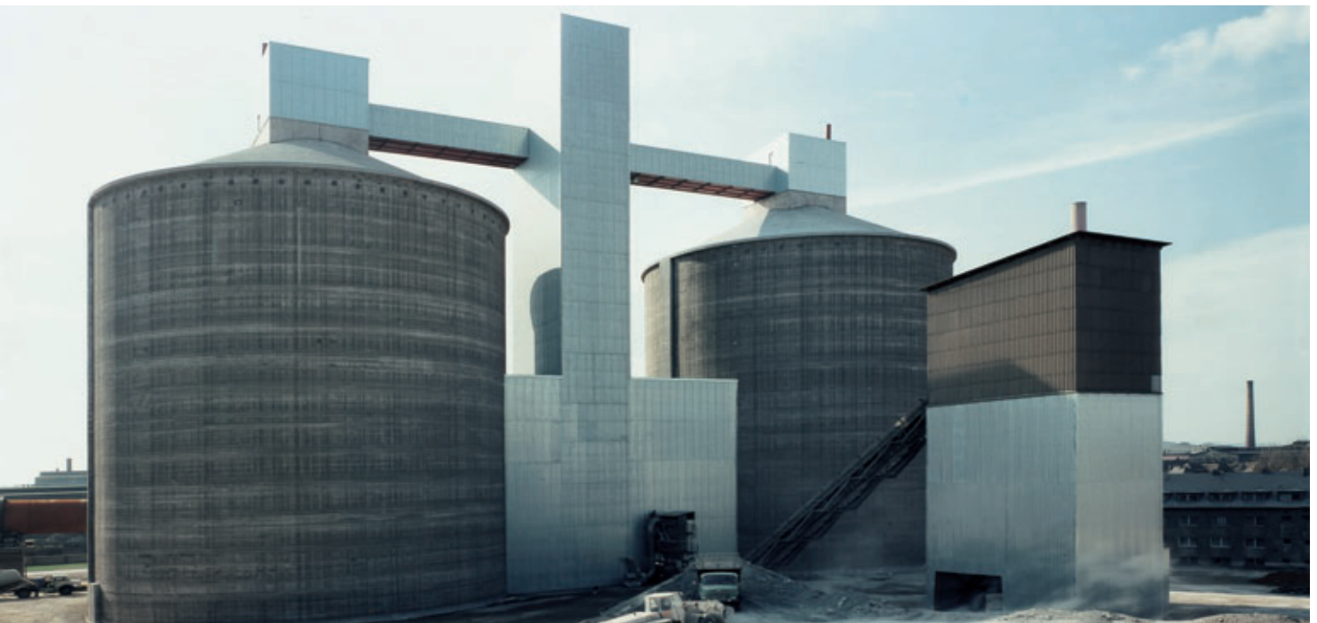
Clinker Silos 2 x 60,000 t
