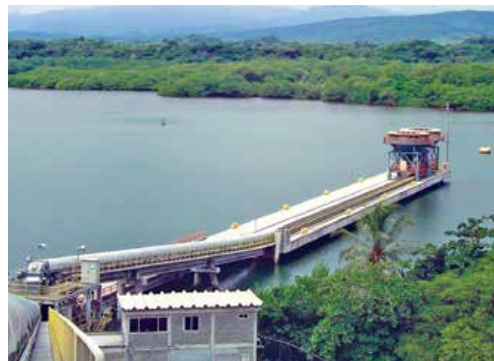
Dedicated concrete jetty with rails for the Eco Hoppers
