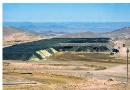
Level plateau stockpile for heap leaching Copper Ore
