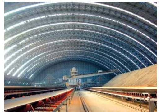
SCHADE blending bed storage with travelling stacker
