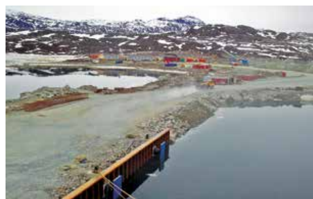
Simple jetty formed in loose rock backfilled
