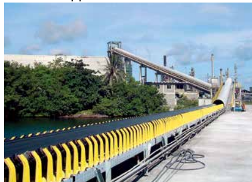
Storage hall linked to jetty by belt conveyor
