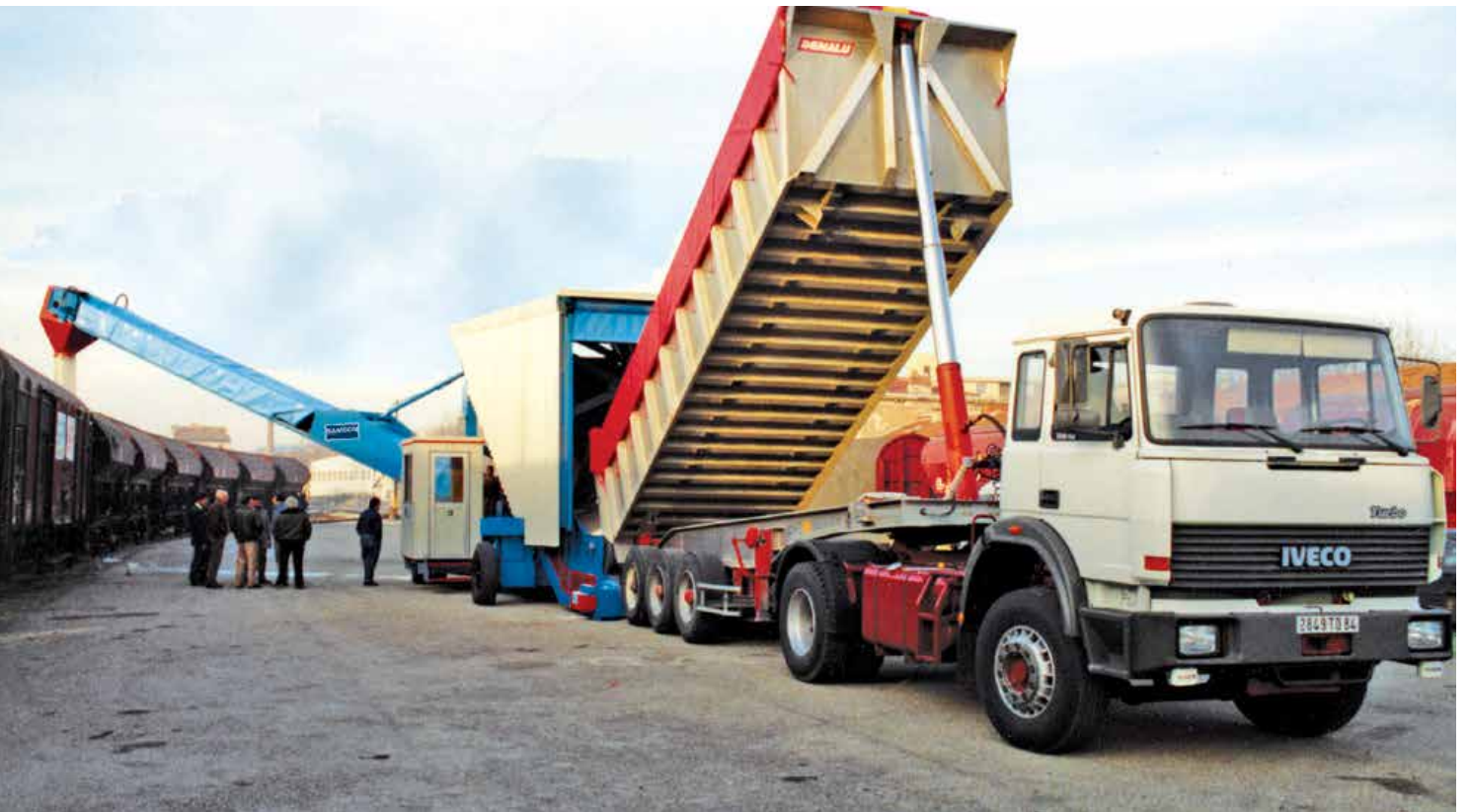
Comprehensive dust enclosures minimise pollution risk allowing controlled loading in this hyper sensitive inner city location
