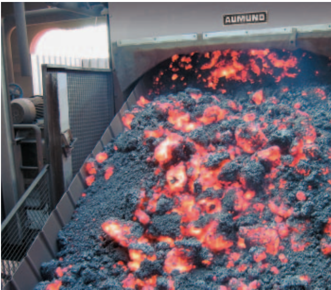
Pan Conveyor, type KZB-S, Sinter plant, Bremen
