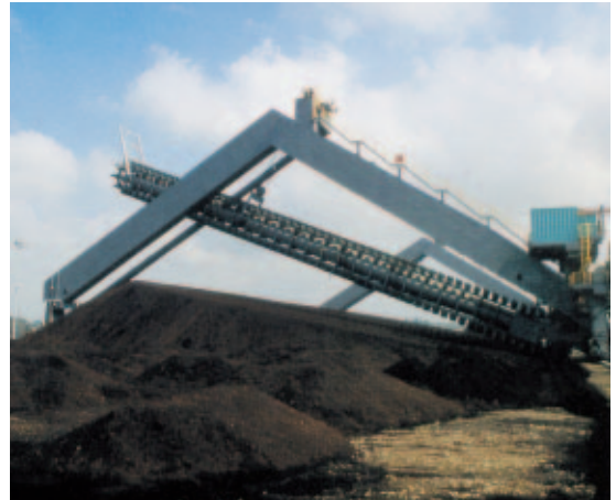
Longitudinal Stockyard with Portal Reclaimers
