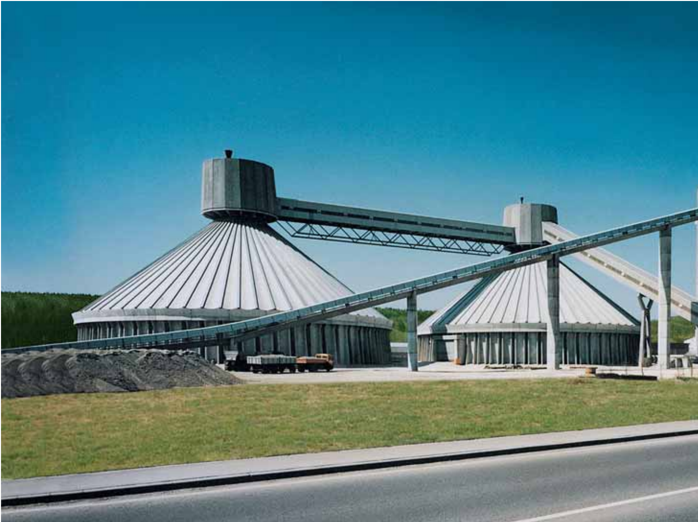
Conveying route with Pan Conveyor KZB
