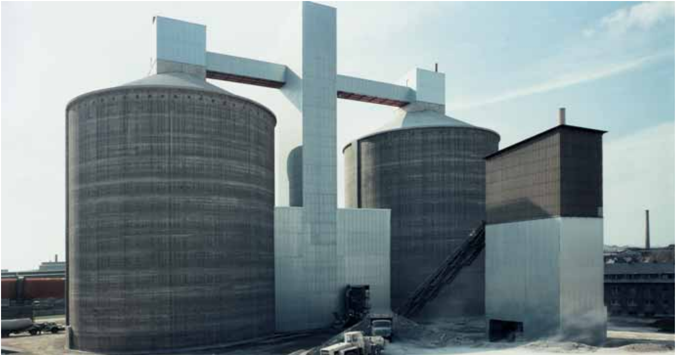
Clinker Silos 2 x 60,000 t
