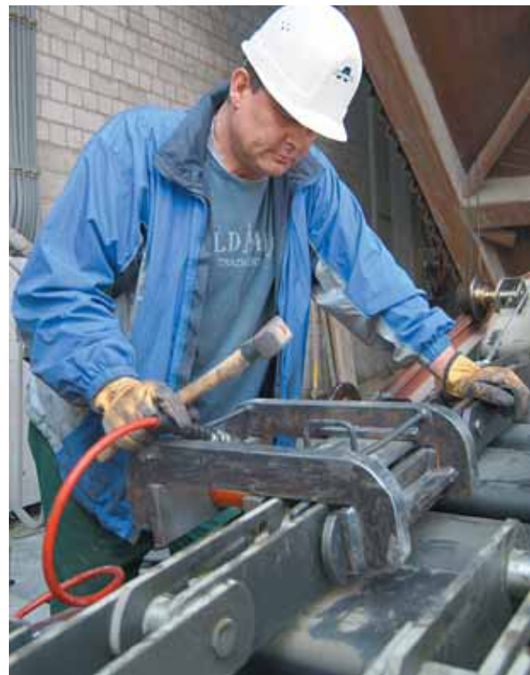
Pre-assembly of chain strands
