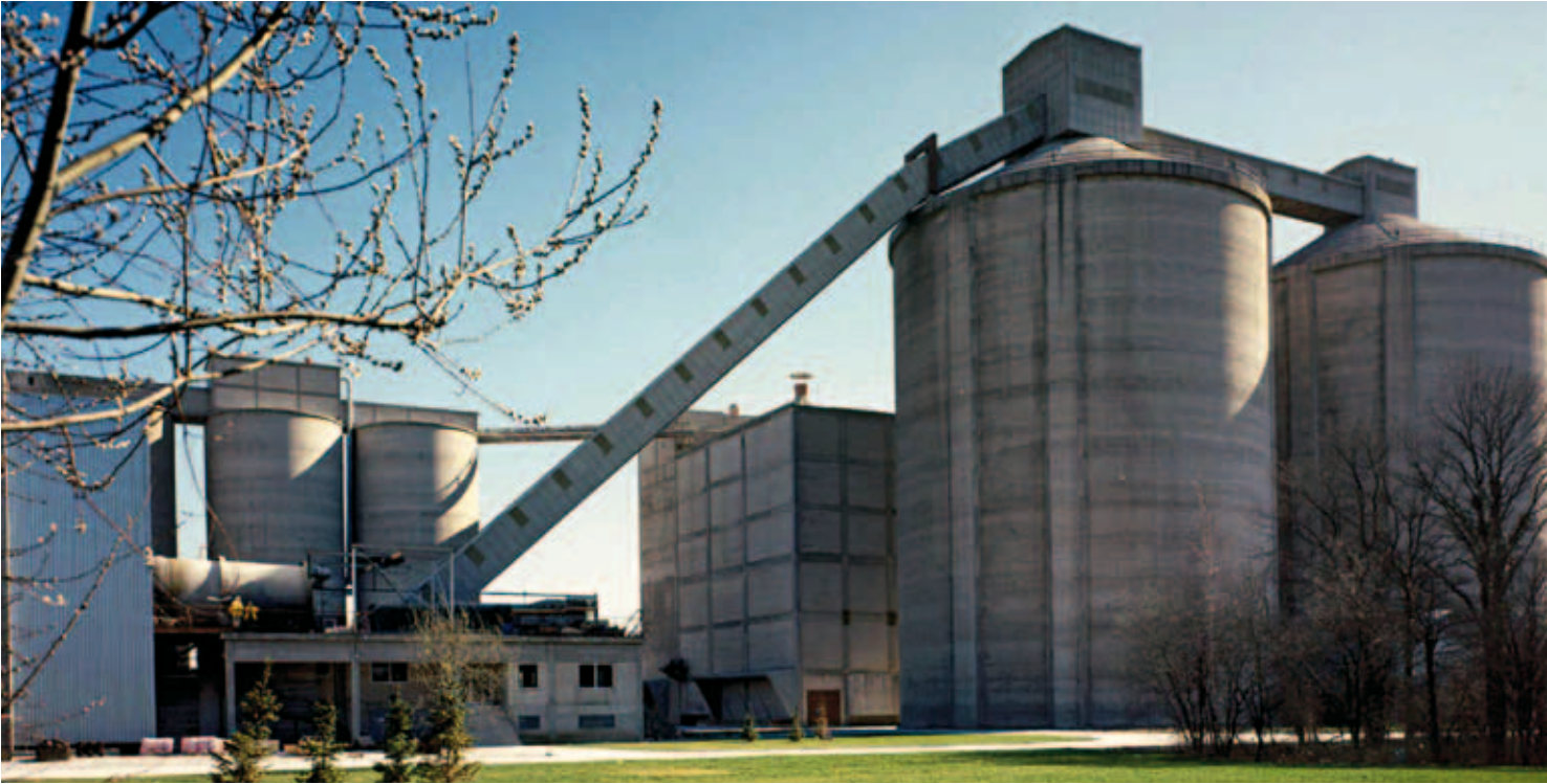
Silo feeding with steep-angle conveyor
