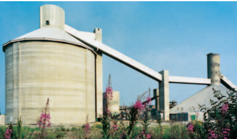
Concrete silo with steel roof
