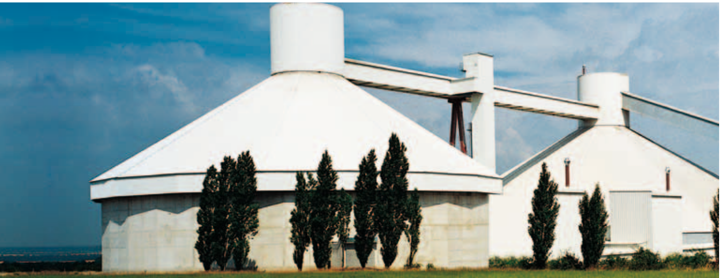
Clinker storage hall with concrete wall and steel roof
