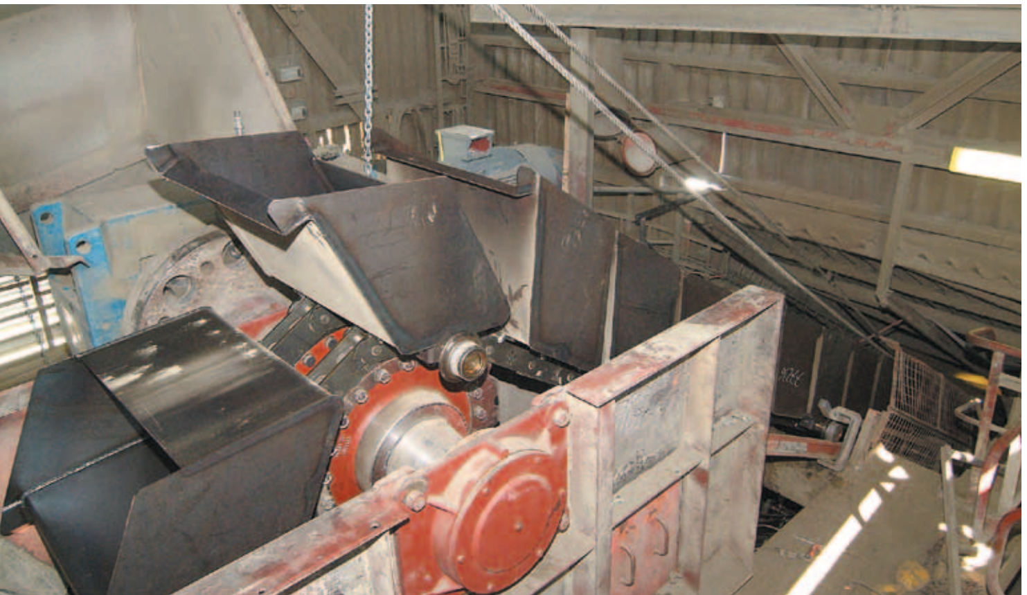
Installation of new bucket strand
