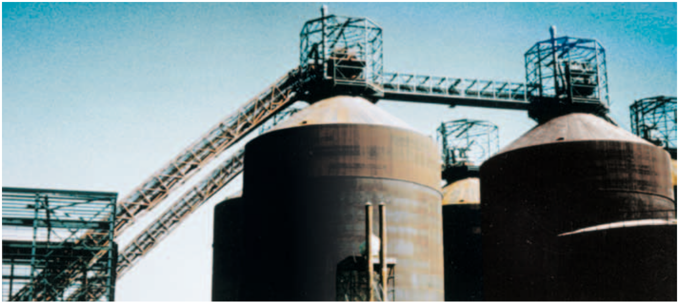
Feeding of steel plate silos
