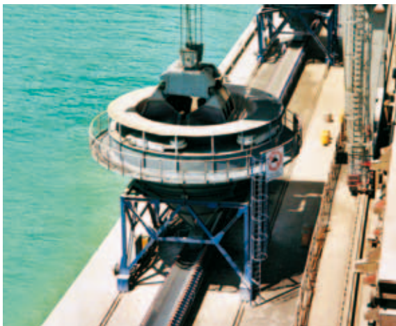
Unloading hoppers for clinker and additives
