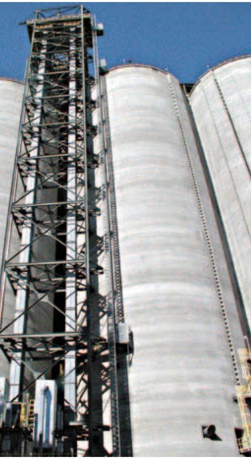
Cement silo feeding
