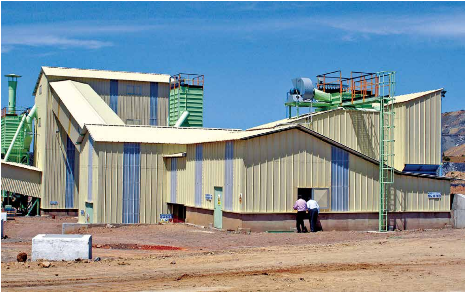
The Samson™ Material Feeder enclosure integrated to a complete coal preparation plant handling ROM material direct from the adjacent open cast mine
