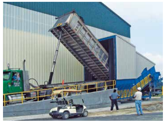
Synthetic Gypsum Intake to Board Plant
