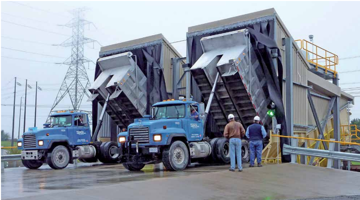
Twin Samson™ Material Feeders receive minus 25 mm Limestone for the Flue Gas De-Sulphurisation system in an US American Power Plant
