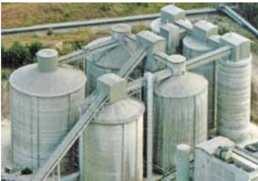
Silo Group for Different Clinker Types
