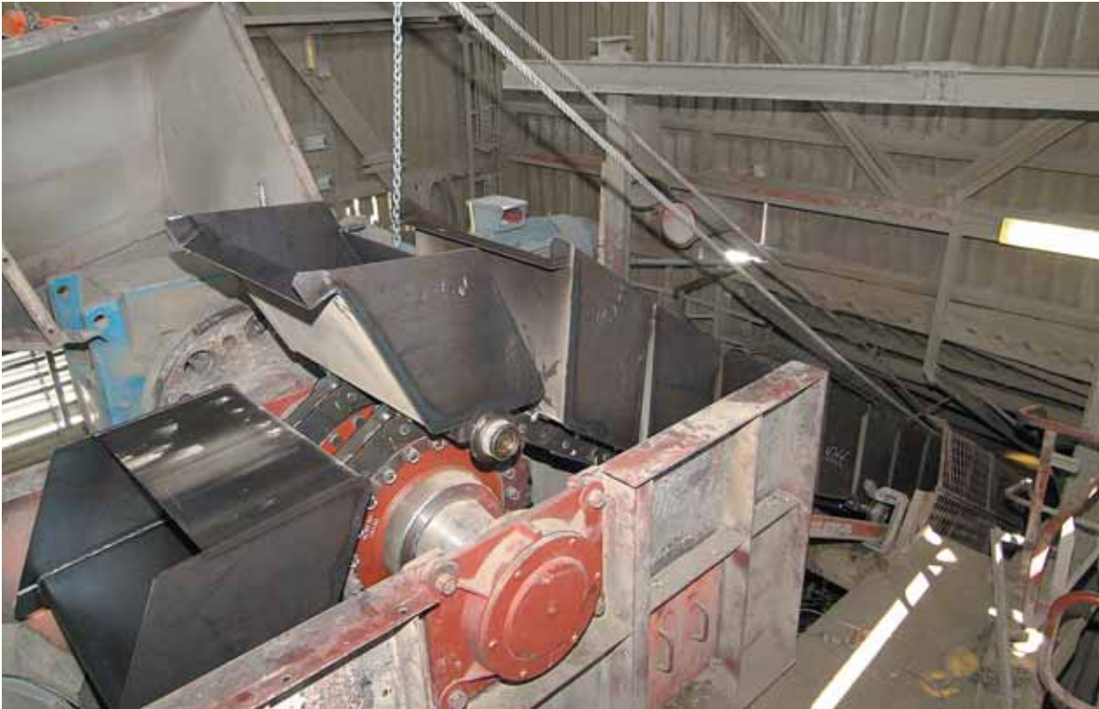
Installation of new bucket strand
