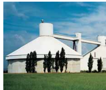
Circular Storage Hall 60,000 t
