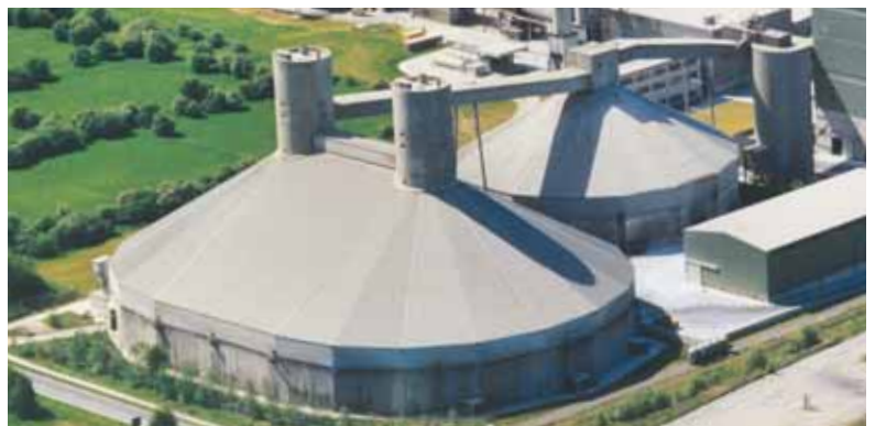
Oval Storage Hall with Two Internal Silos
