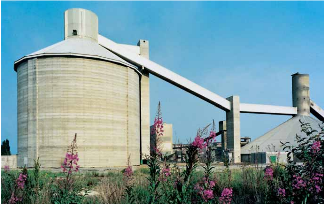
80,000 t Silo with Steel Roof
