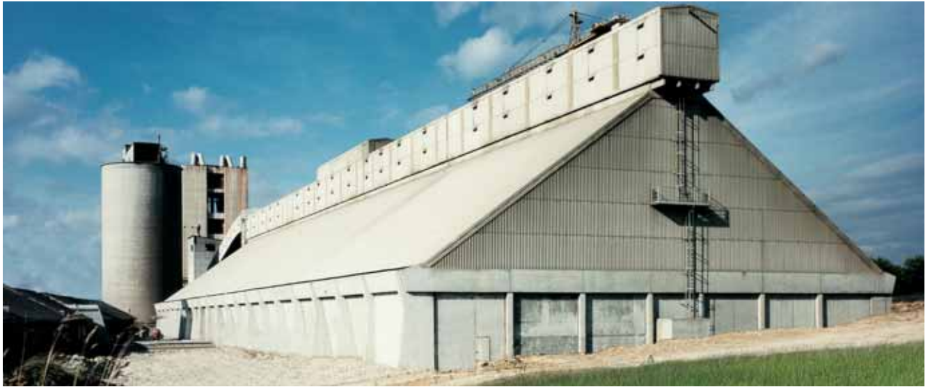
Clinker Storage Hall with Earth Cone
