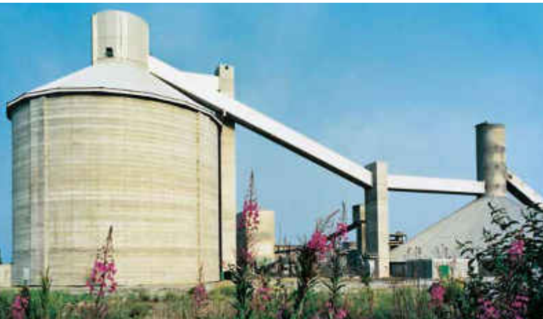
Concrete silo with steel roof
