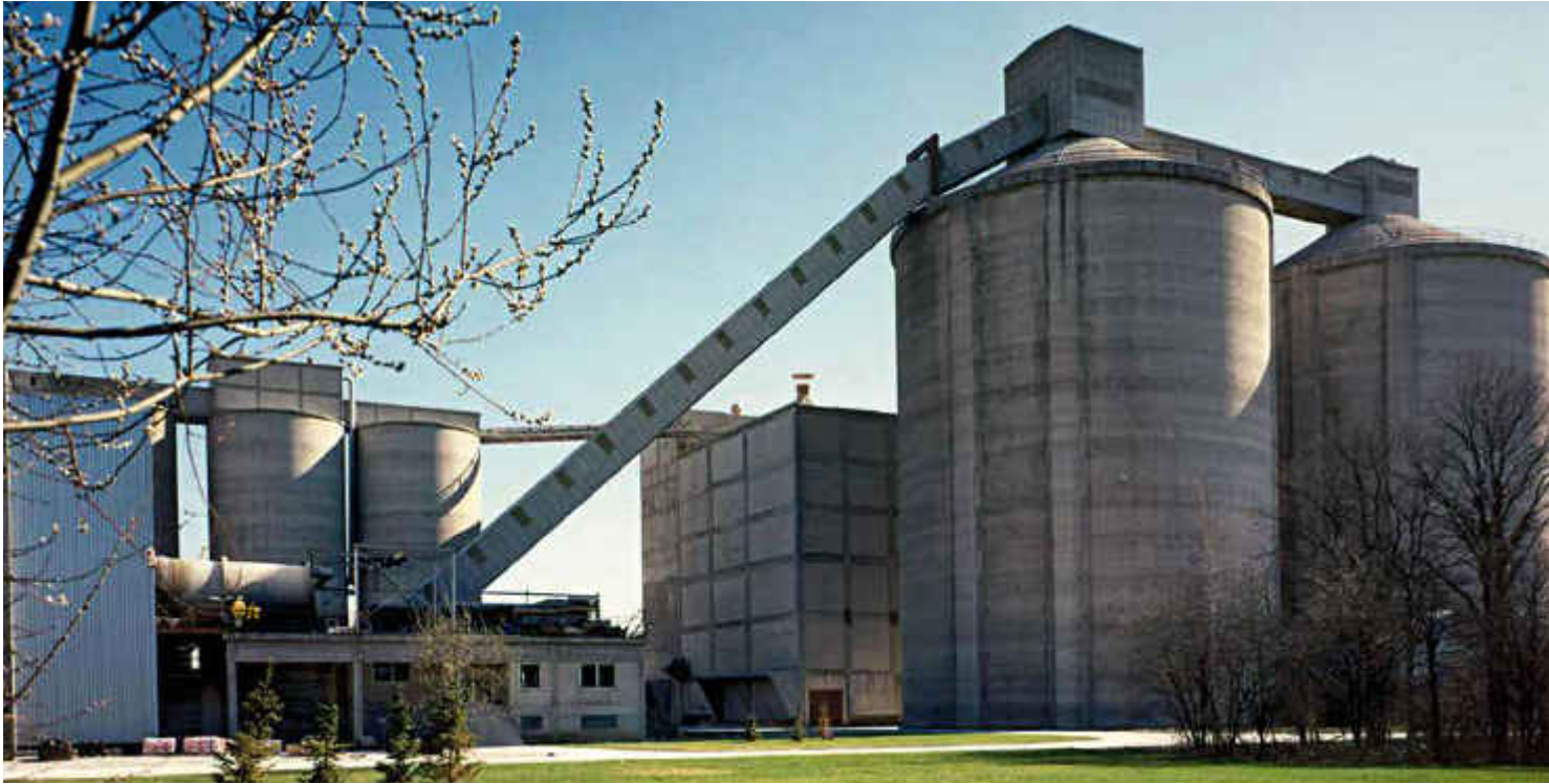
Silo feeding with steep-angle conveyor
