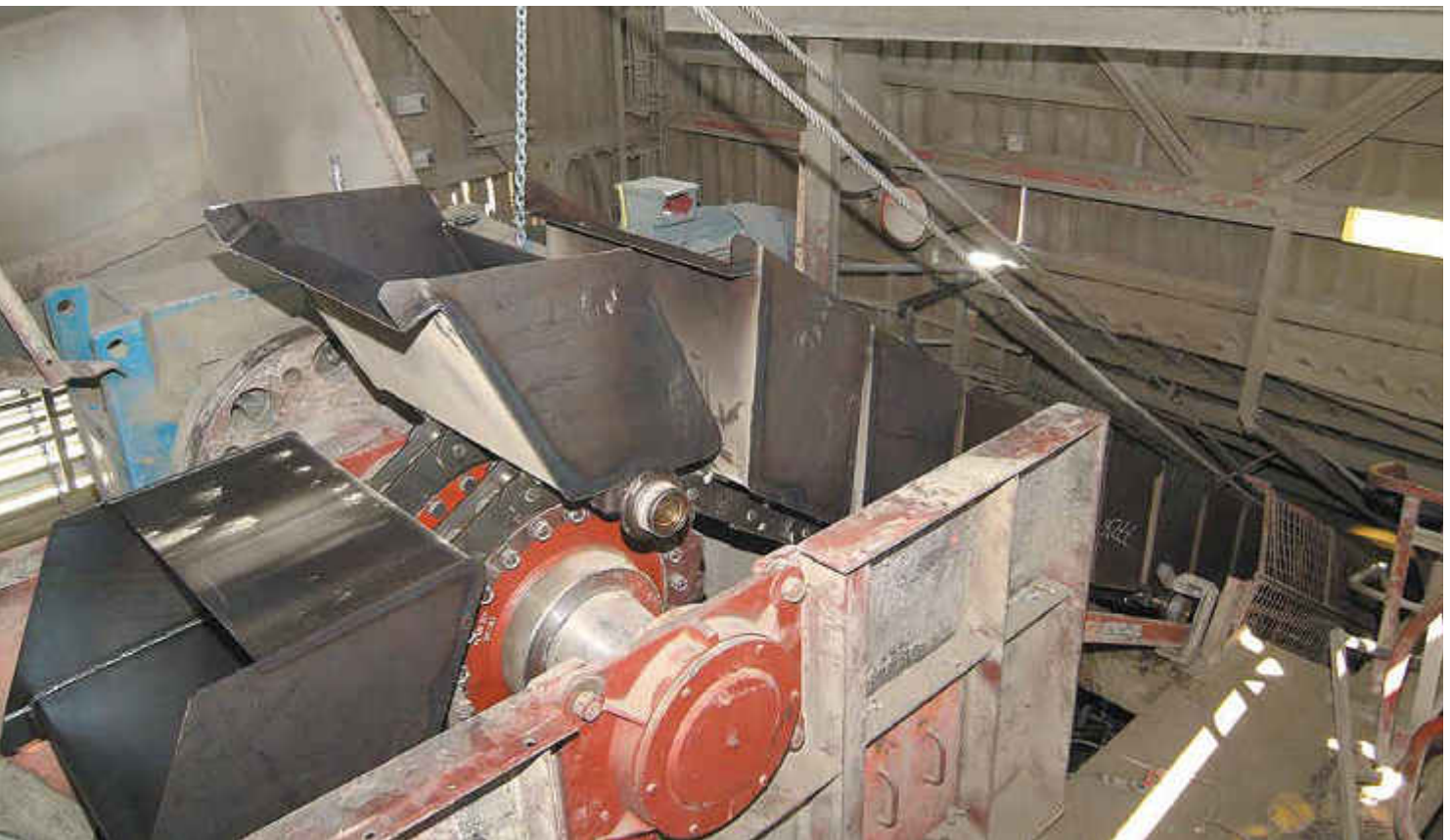
Installation of new bucket strand
