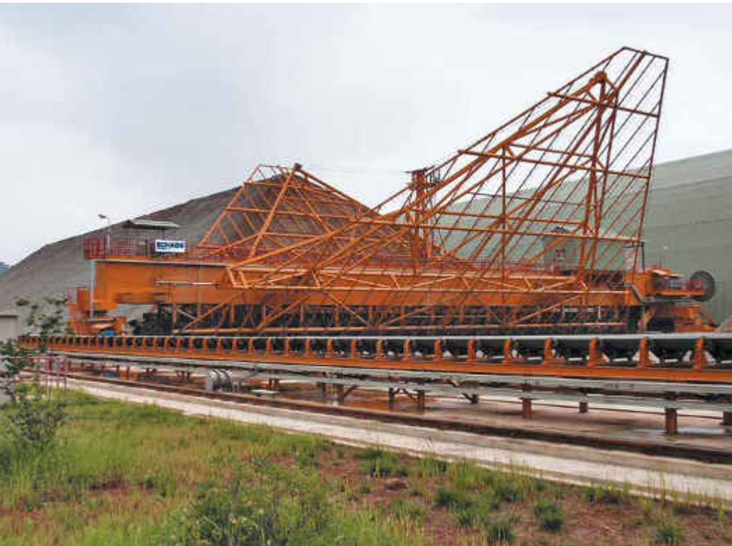
Bridge Scraper Reclaimer for limestone
