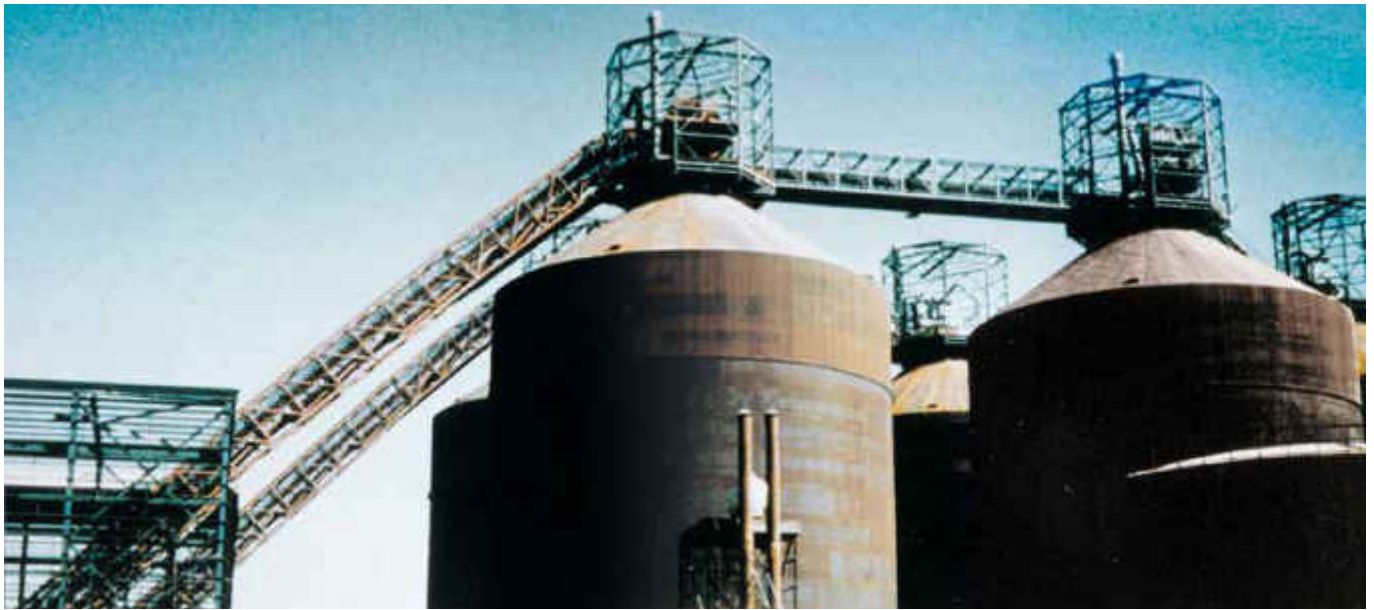
Feeding of steel plate silos
