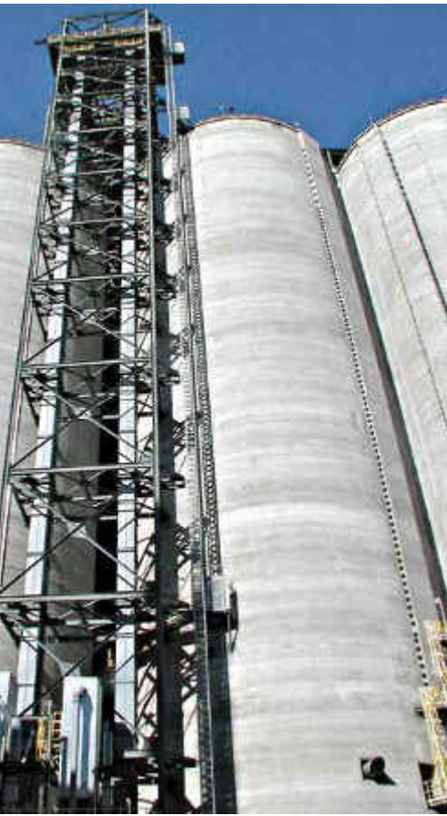
Cement silo feeding
