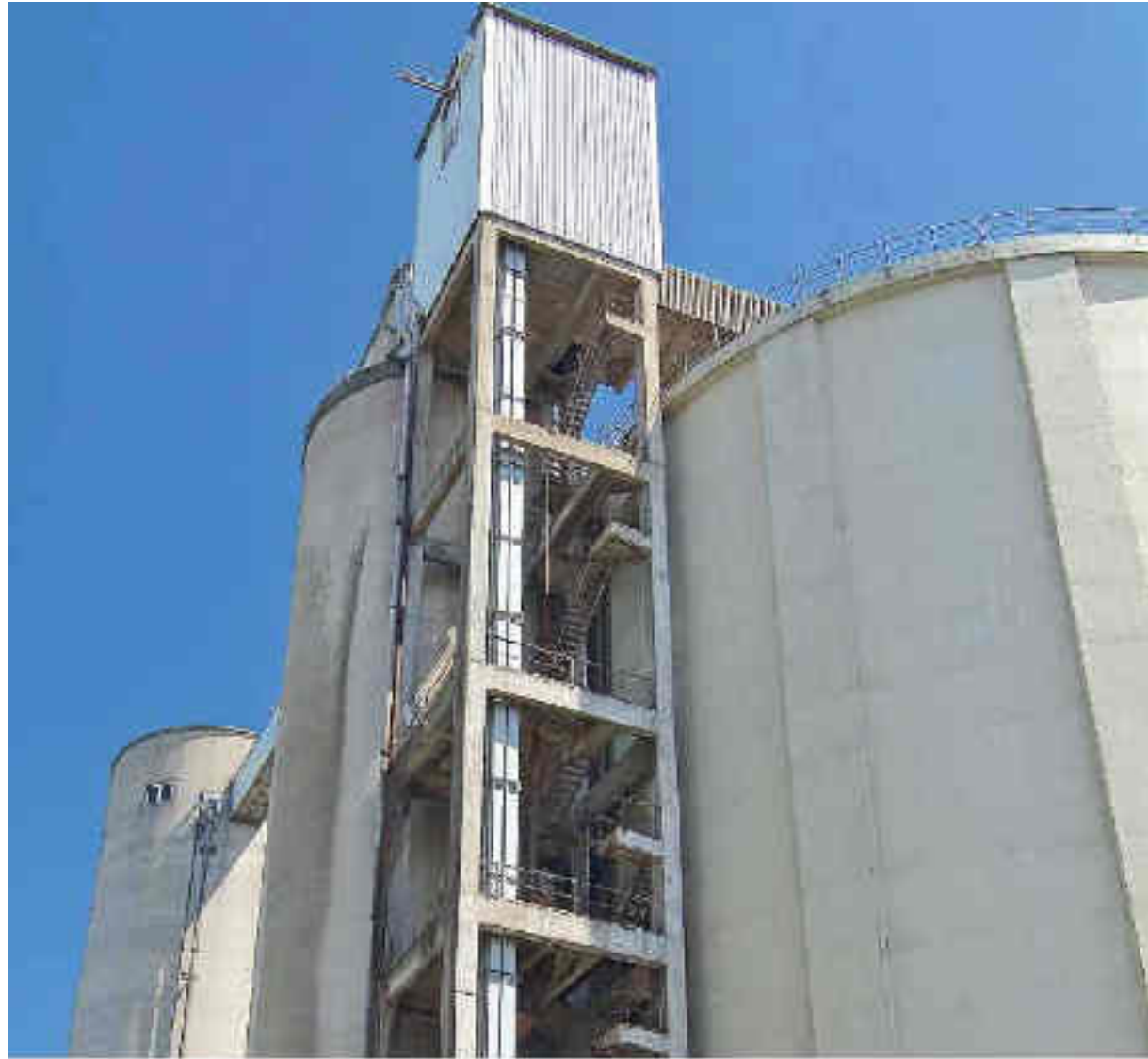
Bucket Elevator for cement silo feeding
