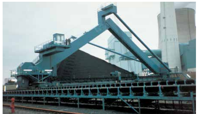
Portal Bridge Reclaimer, 50 m span, 1,225 m 3 /h for combined storage and blending of various coal qualities
