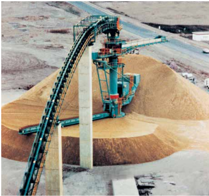
Circular Stacker / Cantilever Scraper Reclaimer, dia 70 m, stacking 1,000 t/h, reclaiming 100 t/h, slag
