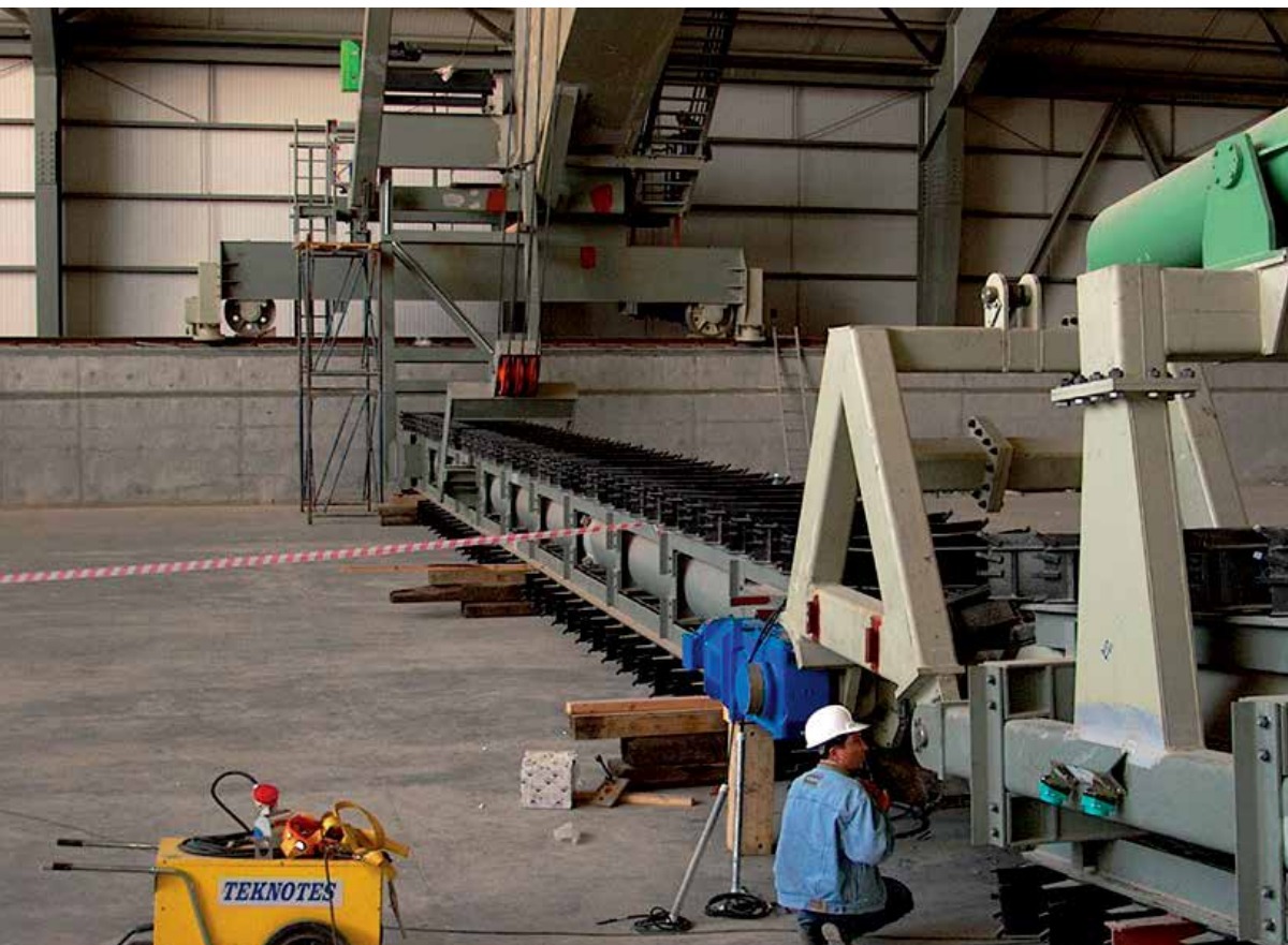
Retrofit situation during capacity increase
