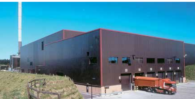
Trucks reverse into closed discharge hall
