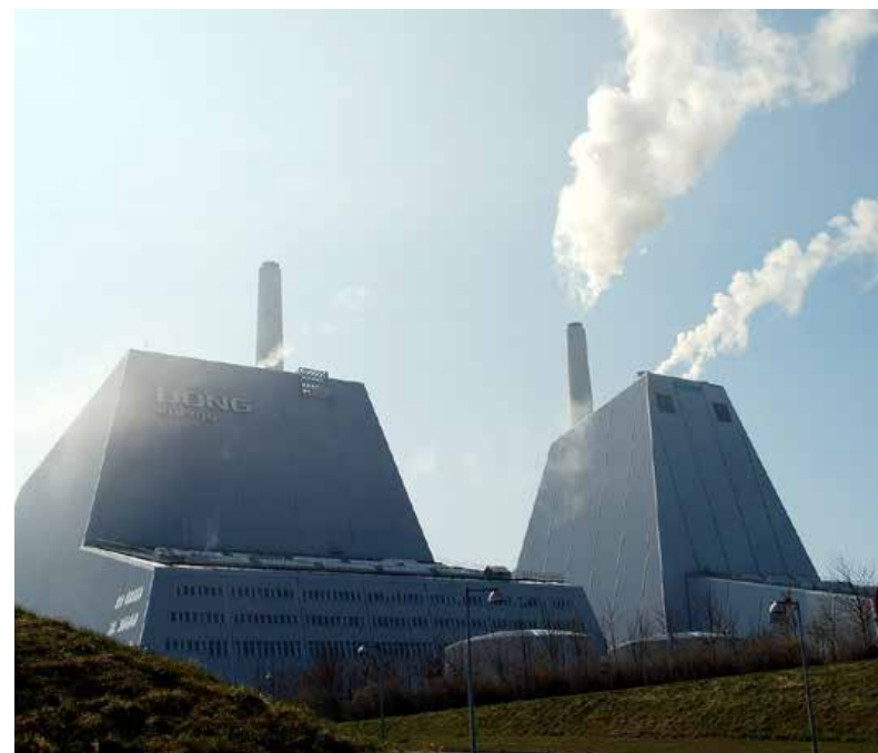
Averdore Multi-Fuel Power Plant in Denmark
