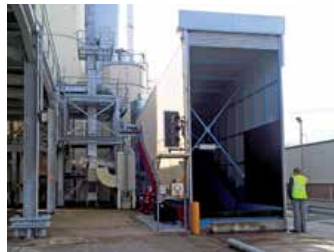
Heineken Brewery Biomass Intake
