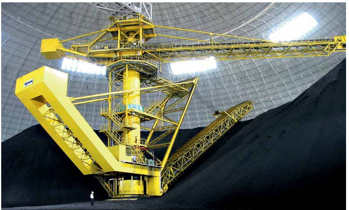
Storage and Reclaim of Iron Ore
