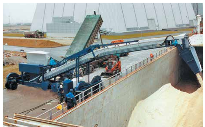
Shiploader – FGD Gypsum
