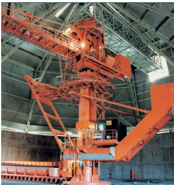
Storage and Reclaim of Iron Ore
