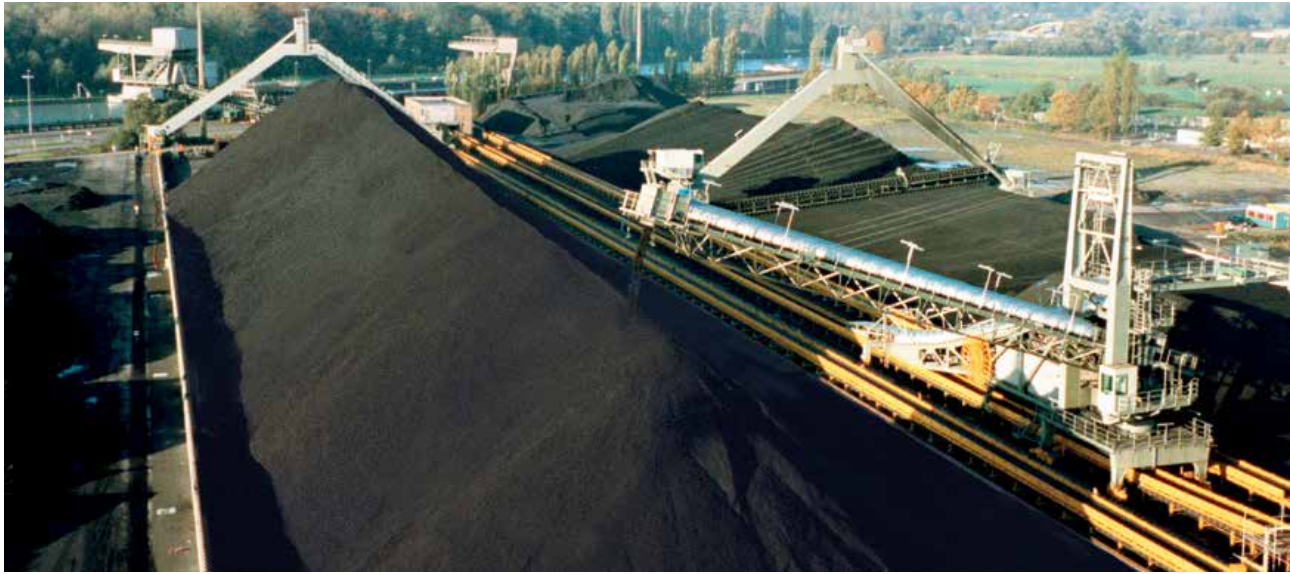
Stockyard with Stacker and Portal Scraper Reclaimers
