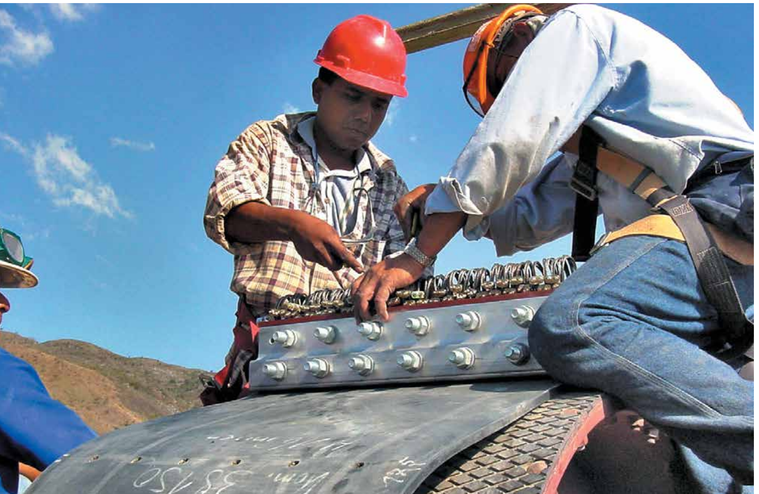
Splicing of steel-reinforced belt
